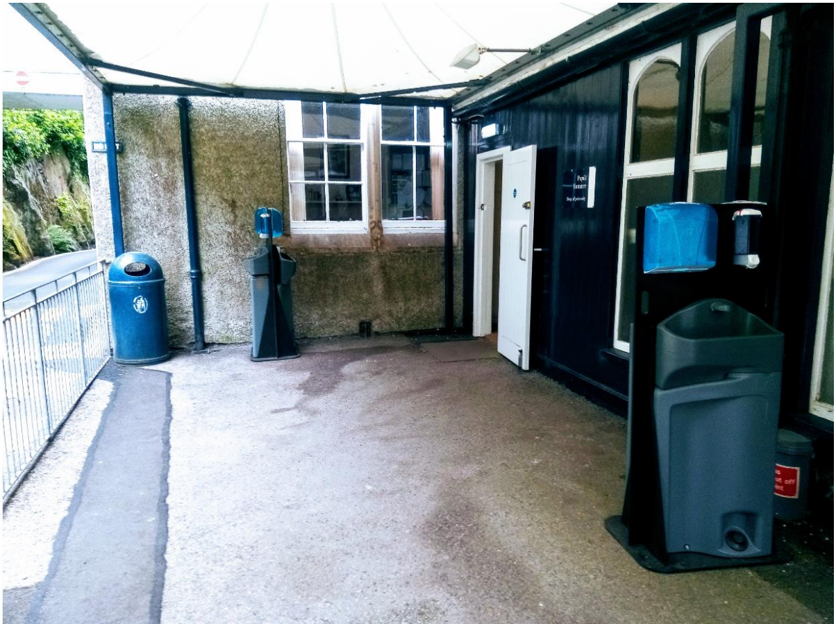
Browhead back door canopy will be used for drop off/ collection of years 7, 8 and 9 and it is equipped with additional handwash facilities.
