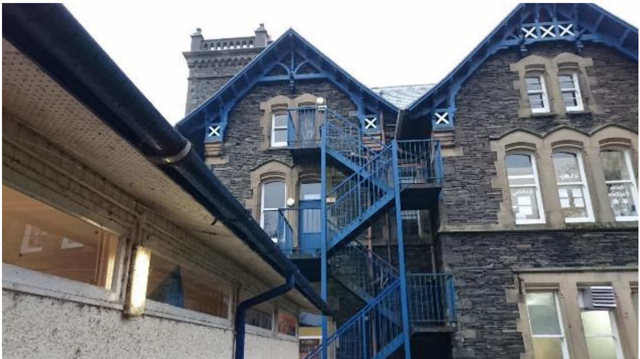
Figure 1 Street view of the premises
